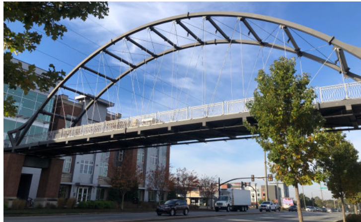
Figure 4: Tied arch Pedestrian Bridge
