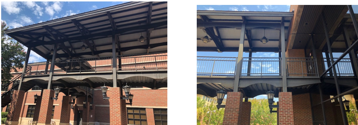
Figure 1: Exterior walkway between two campus buildings
