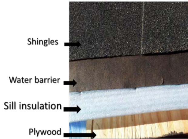
Figure 11: Sill Assembly
