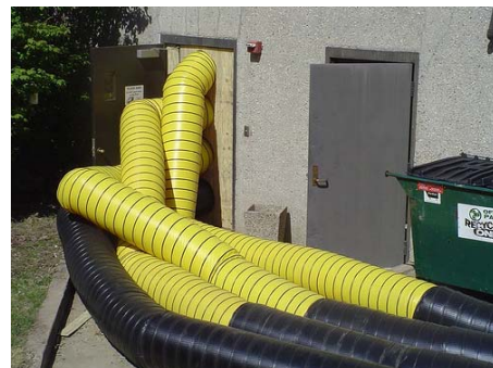
Drying tubes coming out of Wendt Library
