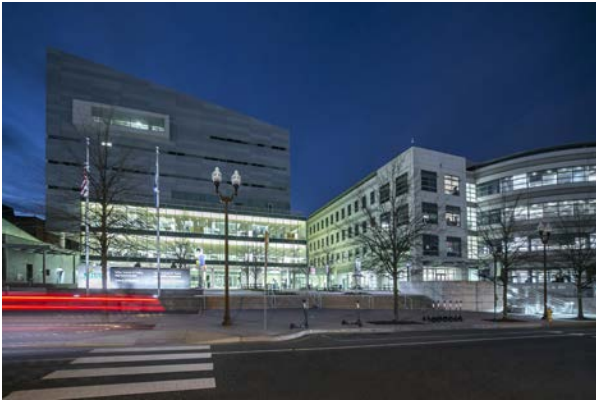
Mason Square at night
