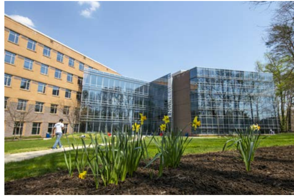
Nguyen Engineering Building on Fairfax Campus
