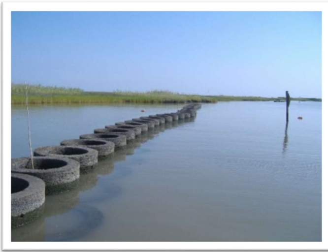
Figure 1. Biofriendly coastal protection devices shortly after emplacement in Gulf Coast marsh area. Rings lock together, are placed parallel to shore, but allow water and nutrient flow through the porous emplacement.
