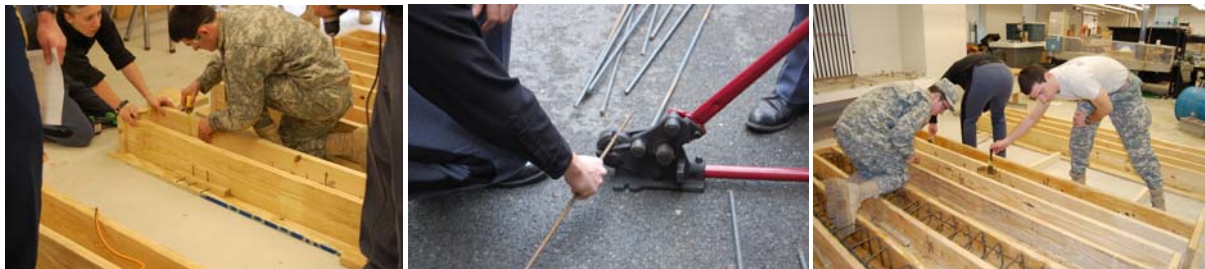
Figure 3 - Construction of the beams.
