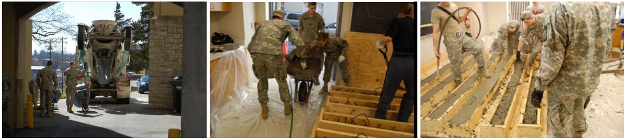
Figure 4 – Placing and curing the beams.
