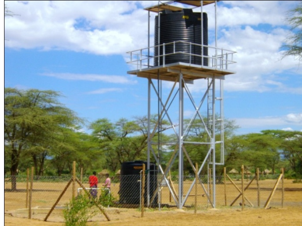
Figure 4. Water Supply Tower at Loongeiwuan
